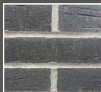
Brick Front Posts
